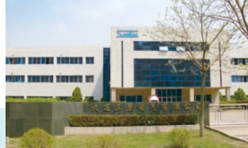
Dalian Sanken Electric Co., Ltd.
