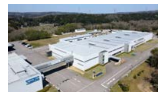
▲ Horimatsu Plant B and the Advanced Technology Promotion Center Total floor space: 10,253.25 m 2
