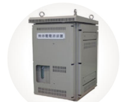
Outdoor power sources for CCTV (crime prevention and security cameras)
